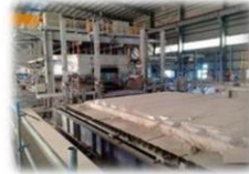
↑ Equipment installation in Vietnam
